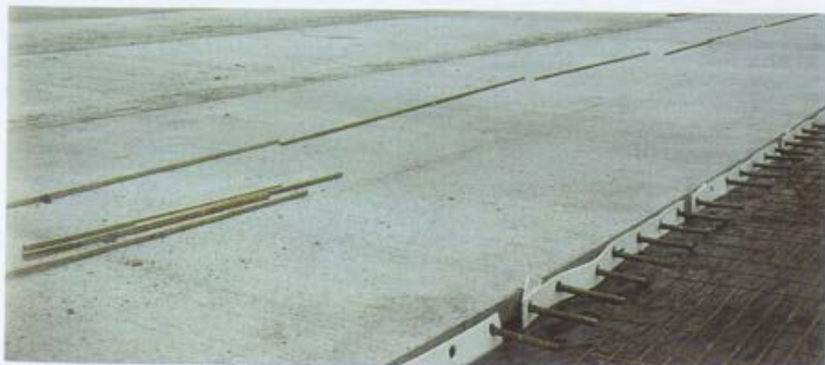
Finished rolled pad – image courtesy of Roller Compacted Concrete
