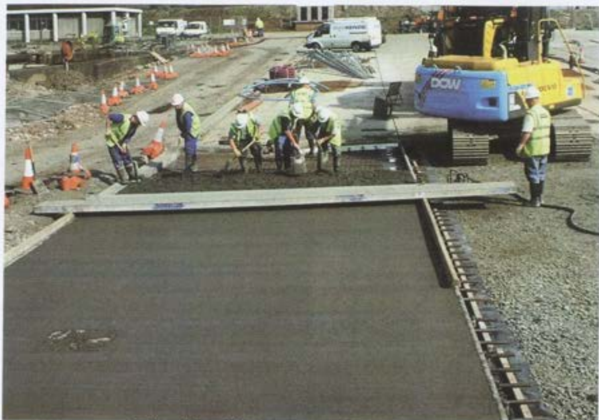
Casting a reinforced slab – image courtesy of Mackenzie Construction
