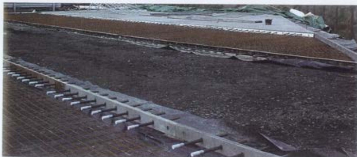
Reinforcement preparation
