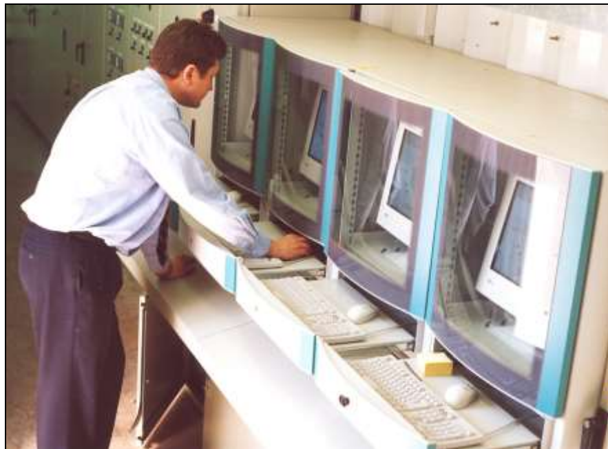
Plate 8: The bank of four PCs, which interface with the PLC systems that run the plant automatically, and are connected to the telemetry systems
