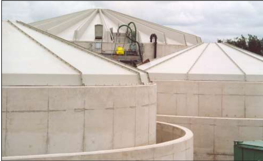
Plate 7: Bundled leachate feed tanks, with one SBR treatment reactor in the background
