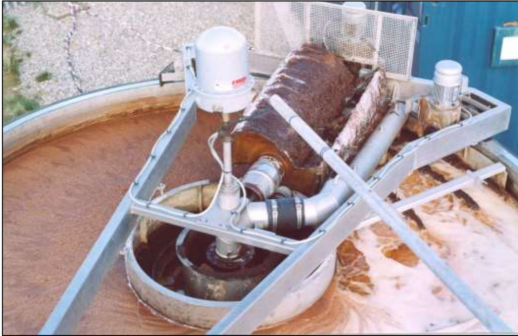
Plate 5: The main DAF tank
