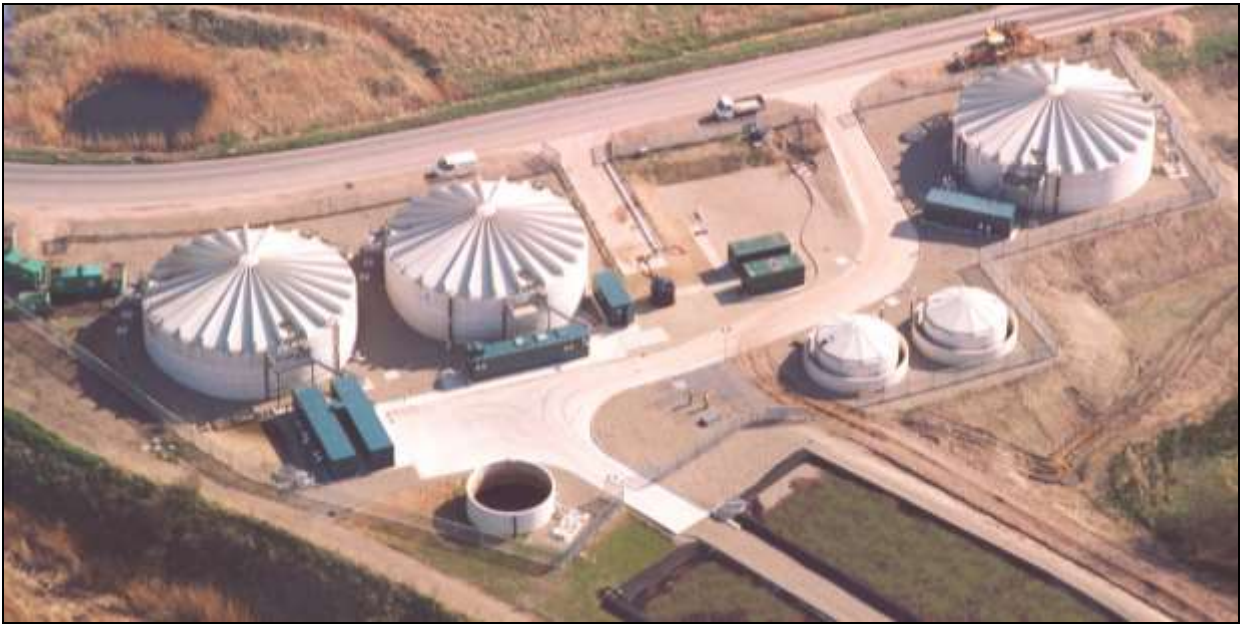
Plate 4: The completed plant, spring 2002, showing the 3 roofed SBR tanks, the twin banded leachate balance tanks, and the effluent balance tank and reed beds
