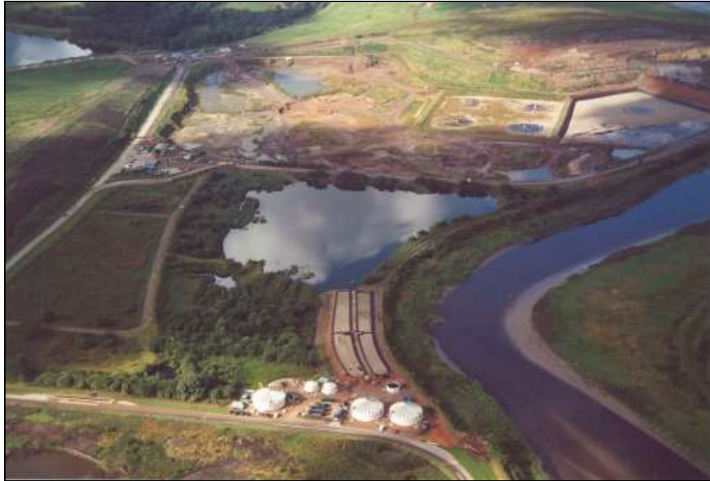
Plate 1: Arpley Landfill, looking due west towards the estuary of the River Mersey showing the leachate treatment plant in centre foreground
