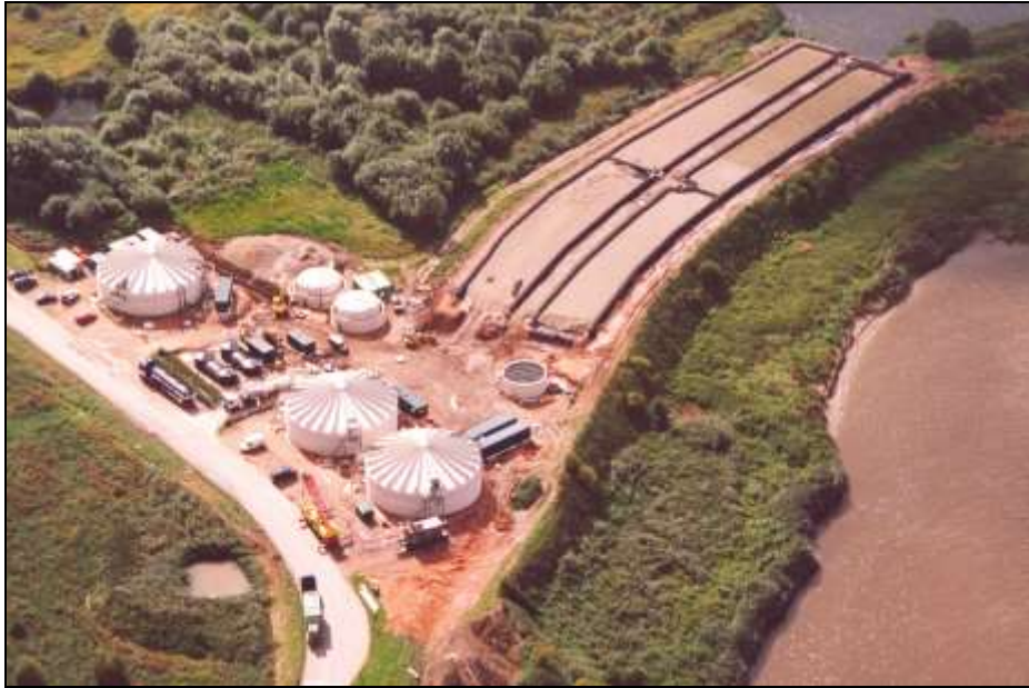
Plate 3: Plant under construction, showing the twin raw leachate balancing tanks, three large SBR tanks, and effluent balance tank and reed beds top right
