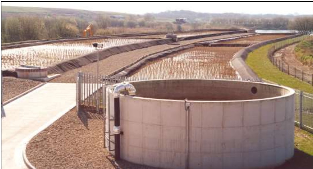
Plate 6: Effluent balance tank, and recently planted reed beds (October 2001)
