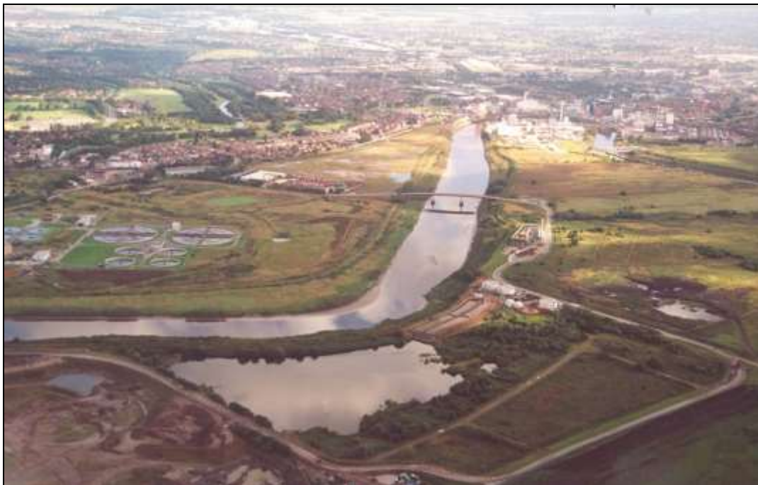
Plate 2: Arpley Leachate Treatment Plant under construction in September 2001, looking north east and showing the landfill (left foreground), Great Sankey STW (left middle distance) and the River Mersey
