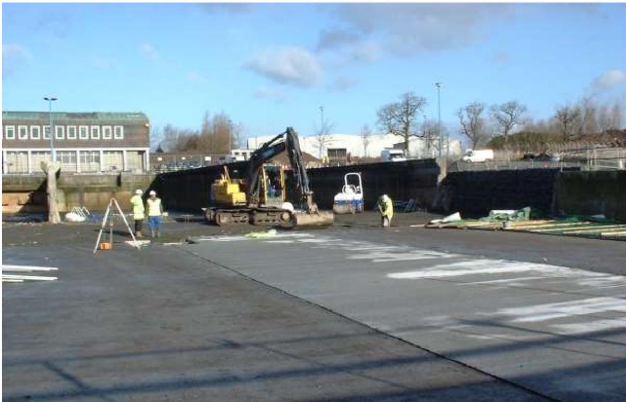
*Plate 4 – View looking north, showing composting plant slab construction in progress in the original Activated Sludge Tanks during February 2005. The Sedimentation tank walls, with ends removed, are visible in the background.*
