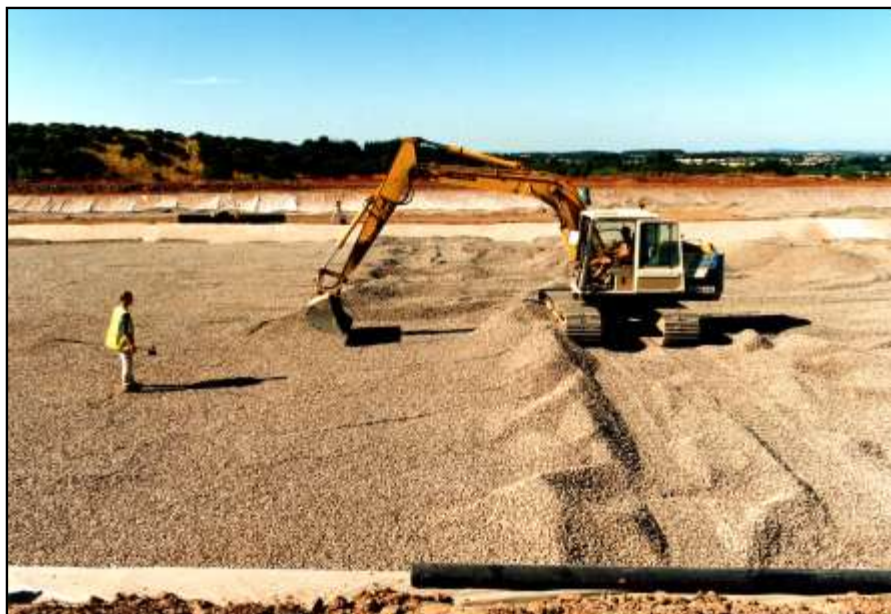
View of the stone levelling operation
