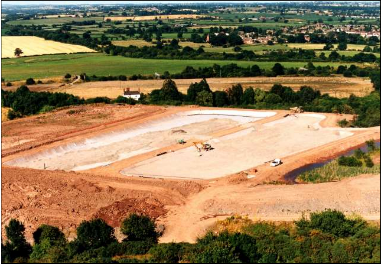
View of the reed beds during construction
