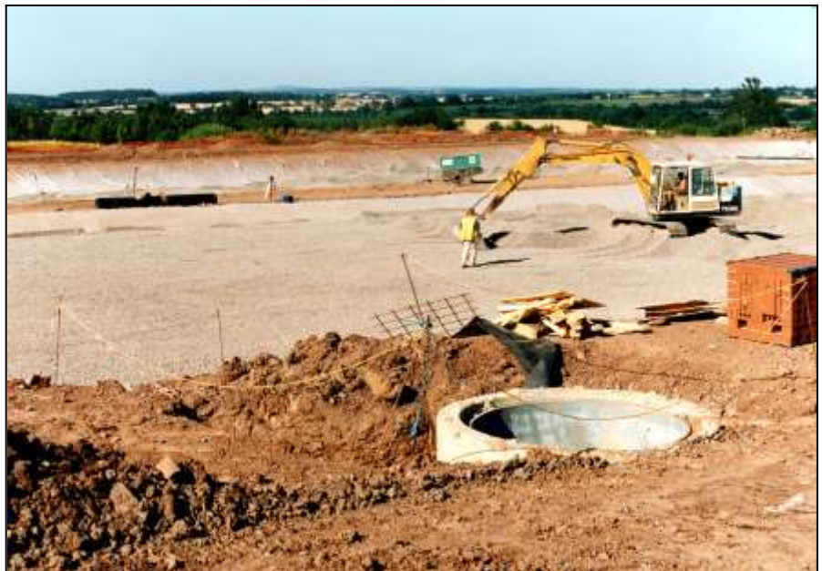
View shows reed bed stone being levelled
